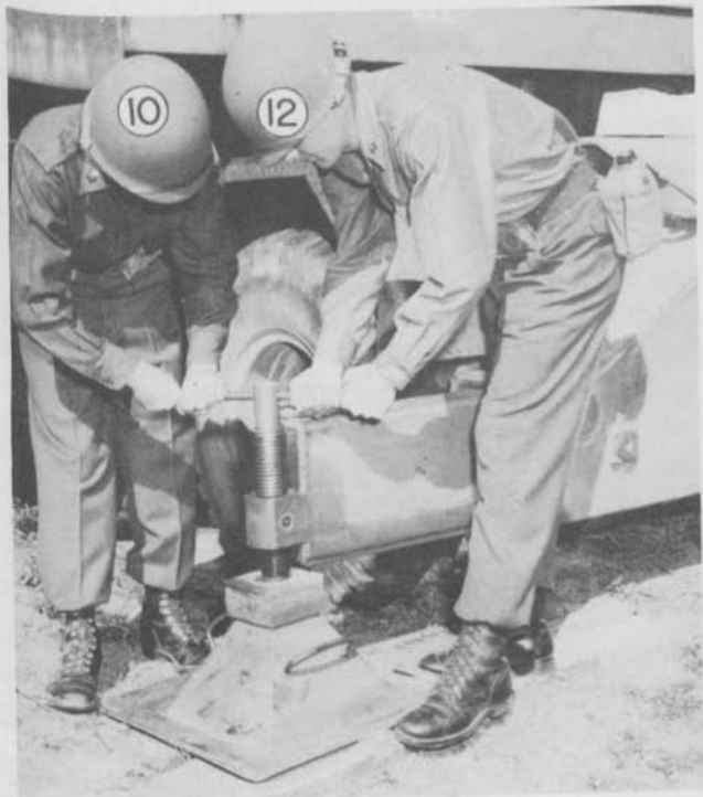
Figure 10. Emplacing outrigger float.
