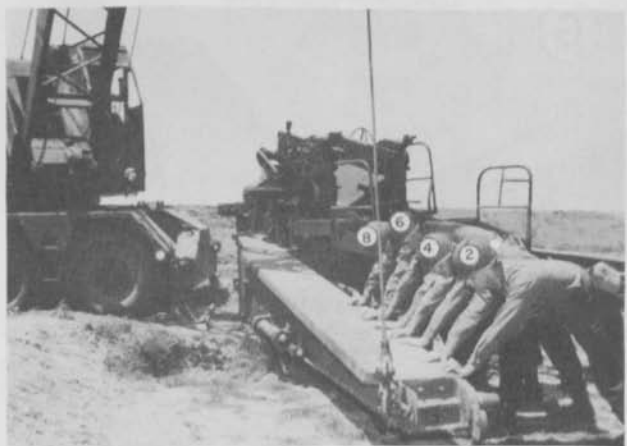
Figure 25. Spreading left trail using single line from the crane.
