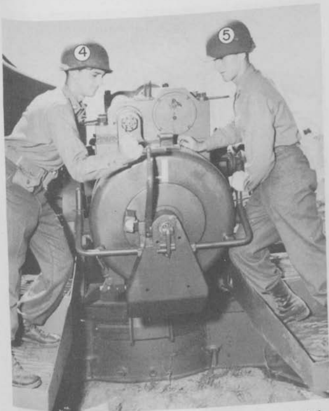
Figure 68. Raising the breech rotating lever to locked position.
