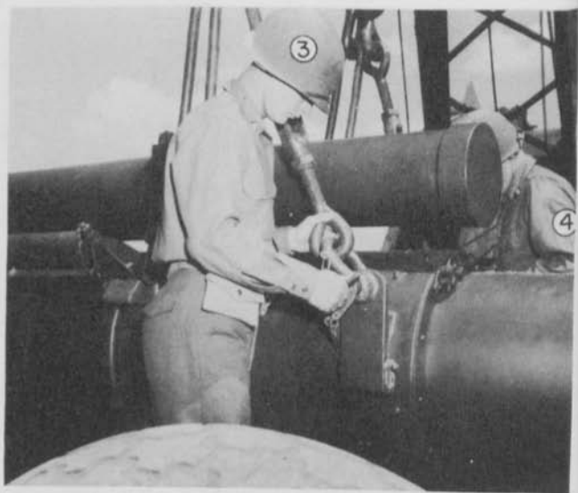
Figure 34. Attaching lifting sling to cradle.
