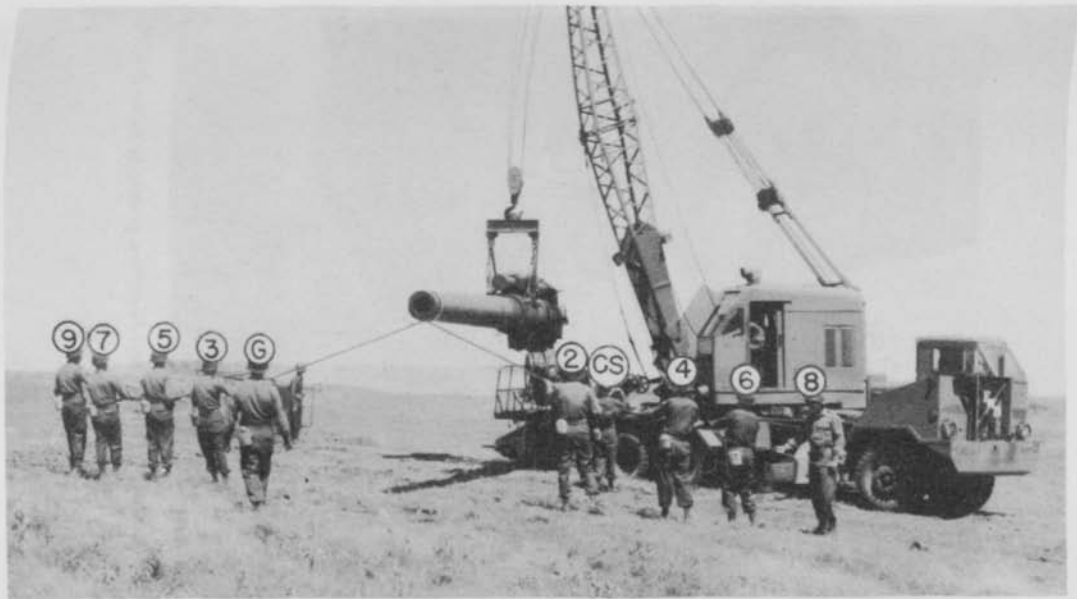
Figure 35. Positioning tube over false cradle.
