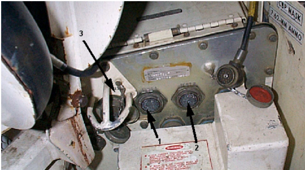
Figure 2-36 M1A1 Trigger and Power Cable Installation
