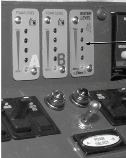
CAB WATER LEVEL GAUGE
