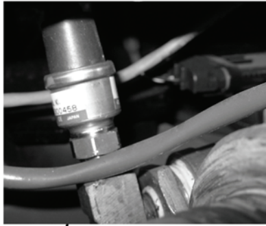
NO. 4 PASSENGER SIDE PRESSURE TRANSDUCER
