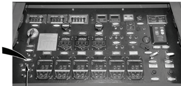
FOAM TANK SWITCH
